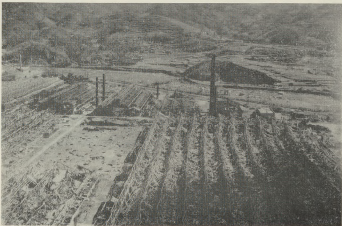
Photo 23. 4500 feet from GZ. Aerial view east.
